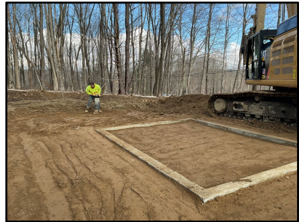
Backfilling/Compaction of Building Foundation
