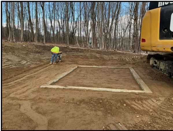
Backfilling/Compaction of Building Foundation
