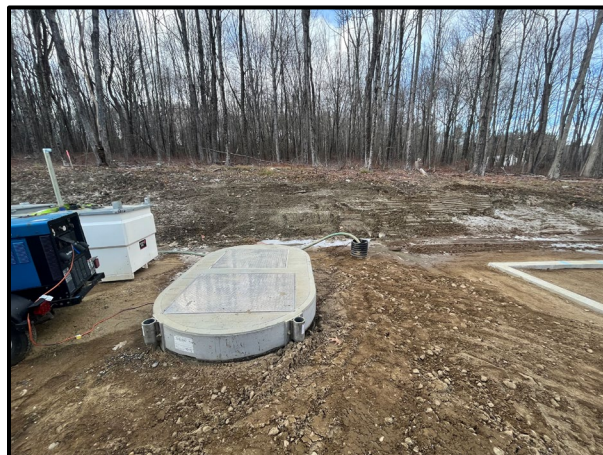
Backfilled Wetwell/Valve Vault Excavation
