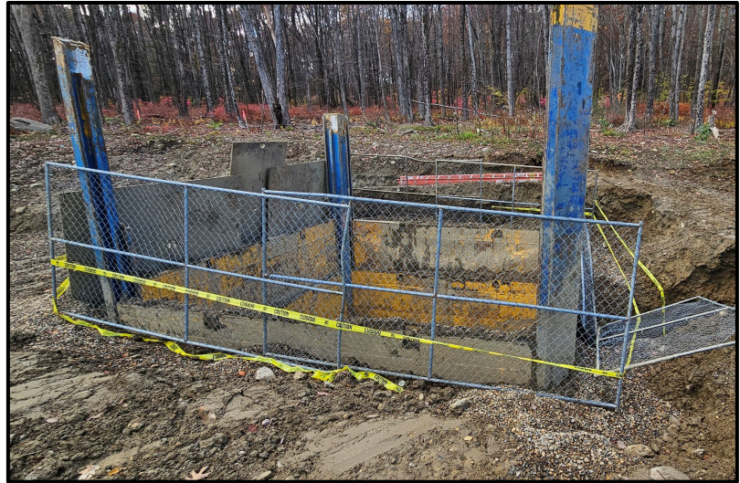
Excavated Wetwell Pit (Water to be Pumped Out Next Week)
