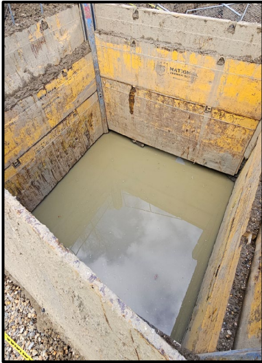
Excavated Wetwell Pit (Water to be Pumped Out Next Week)
