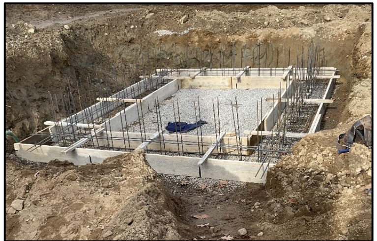
Foundation Footing Forms/Rebar
