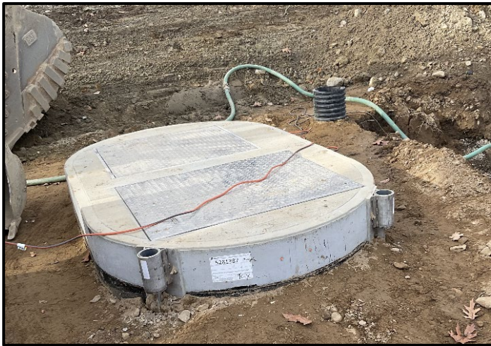
Backfilled Wetwell/Valve Vault
