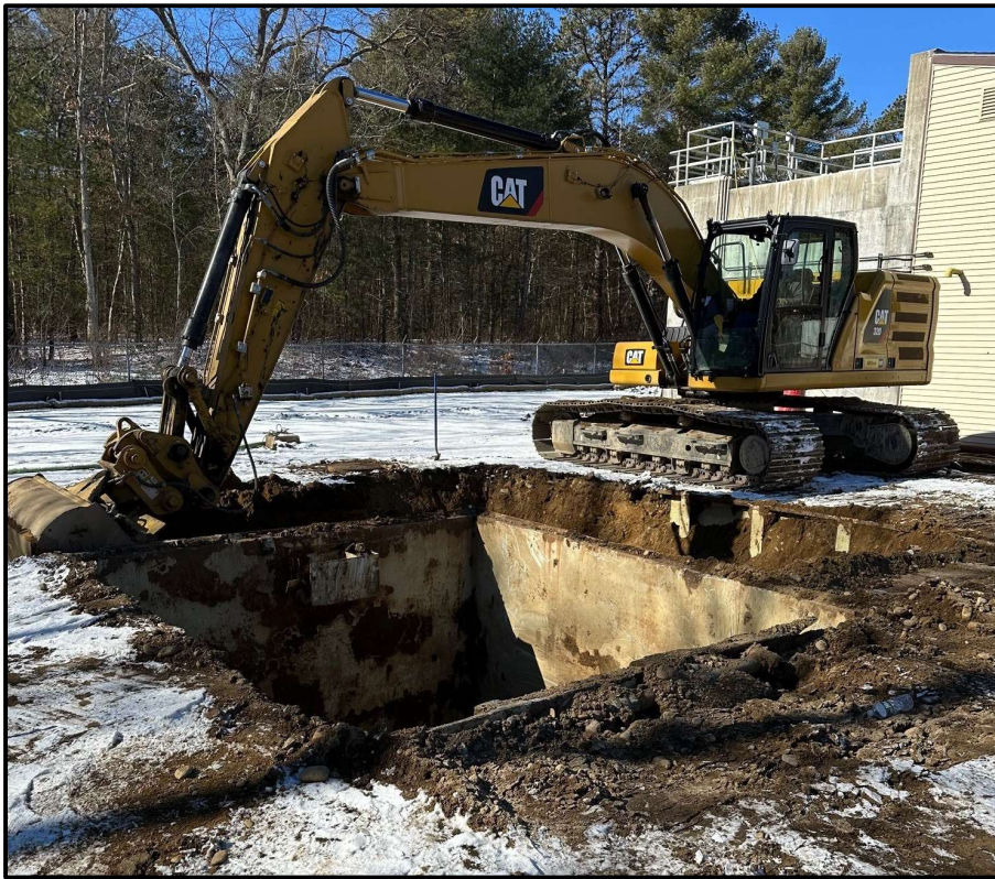
Excavation and Demolition of Existing/Abandoned Clarifier Tanks
