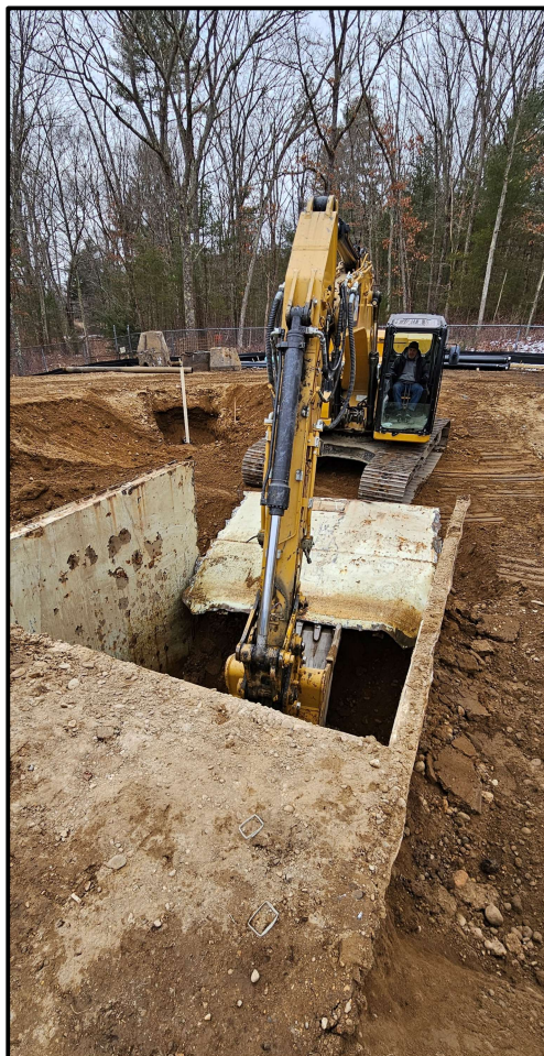
Demolition of Existing/Abandoned Clarifier Tanks and Effluent Manholes
