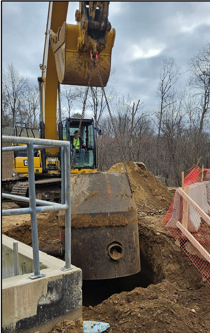
Demolition of Existing Effluent Manhole
