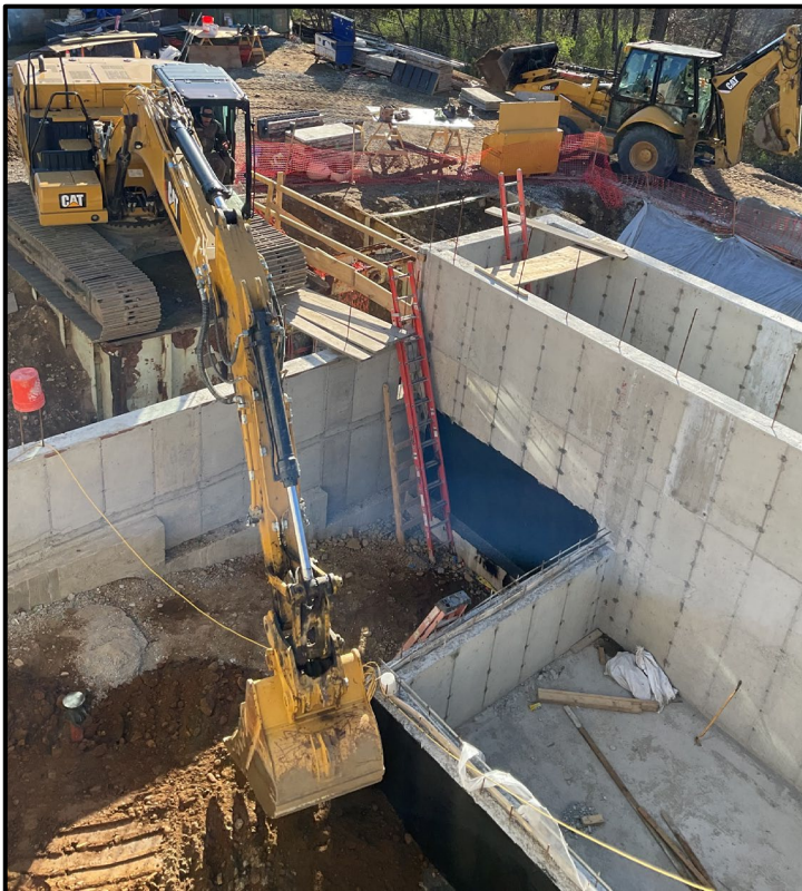
Bringing Fill up to Grade for New Slab
