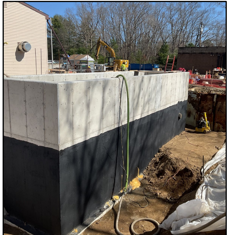
Sealed Clearwell Walls Following Successful Water Tightness Test
