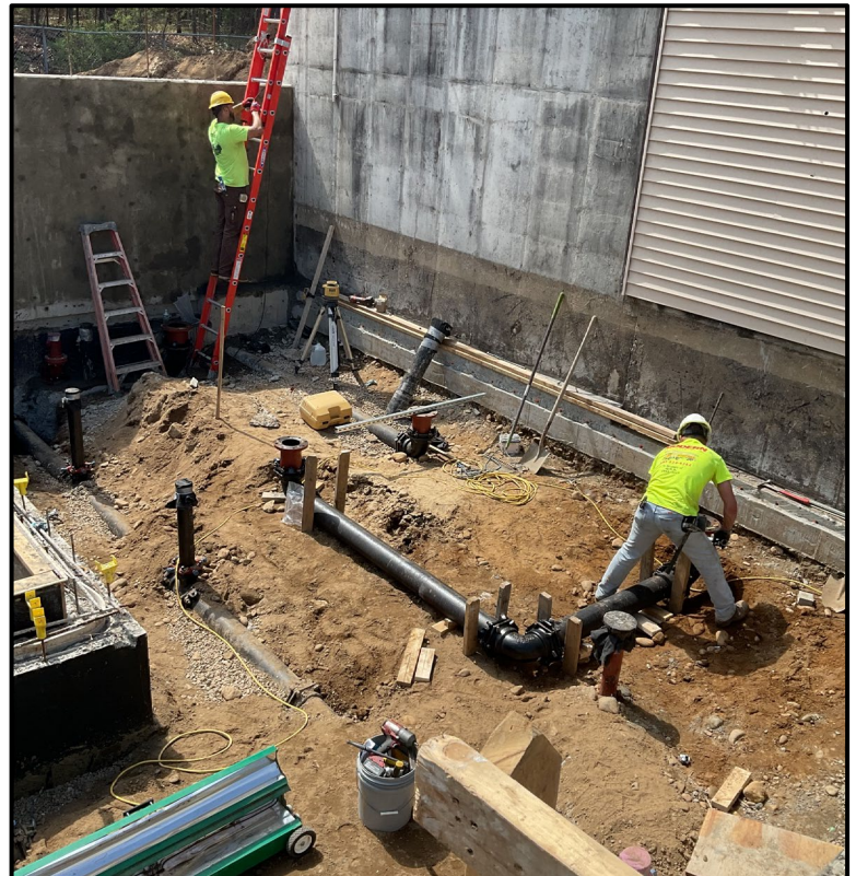
Installation of UV Bypass Piping and Conduit Work
